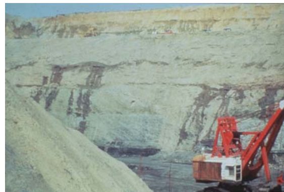
Figure 3. Seepage from Upper Aquifer Materials on an Excavation Face (Photo compliment of Dr. Tim Kimmis, Midwest GeoSciences Group)
